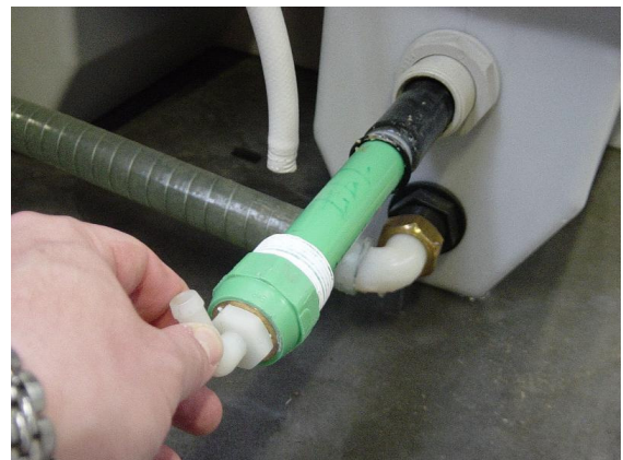
Removing the aerator unit
