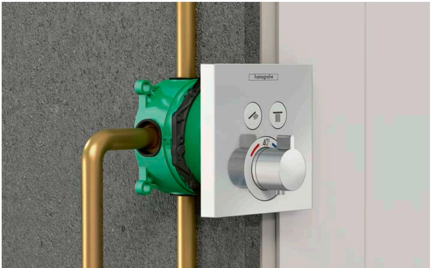
**Concealed installation:** The basic set disappears completely into the wall. Mixers and shower finish sets from various ranges can be fitted to it.
