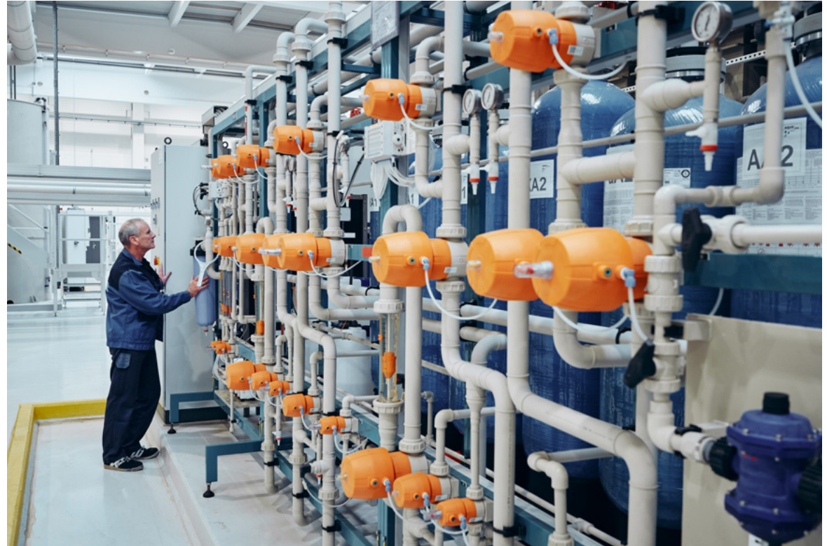
The water treatment system in our Offenburg plastic electroplating facility, a so-called ion exchanger, helps to use water sustainably.
