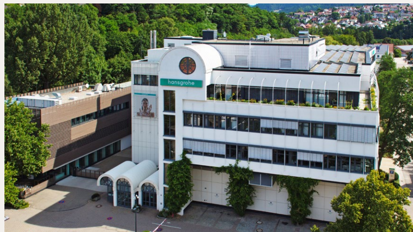
The Hansgrohe Group's headquarters are located in the center of the small Black Forest town of Schiltach.
