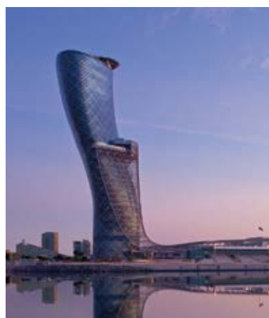
Hotel Hyatt Capital Gate, Abu Dhabi: głowica prysznicowa Raindance® S 240 Air.
